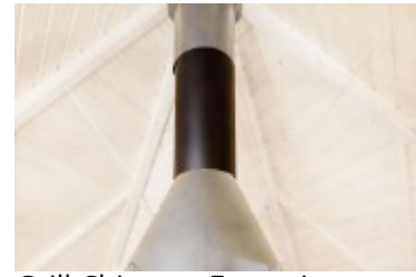
Grill Chimney Extension
