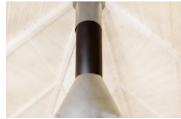
Grill Chimney Extension
