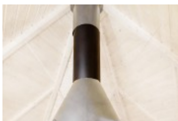
Grill Chimney Extension
