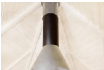
Grill Chimney Extension
