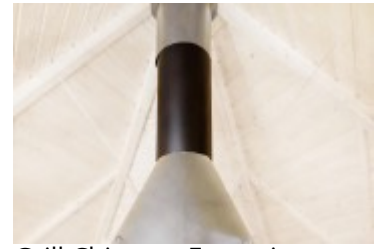
Grill Chimney Extension
