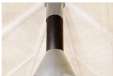
Grill Chimney Extension
