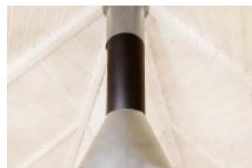
Grill Chimney Extension
