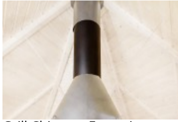
Grill Chimney Extension
