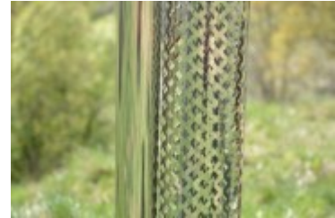
Metal safety fence for heater chimney
