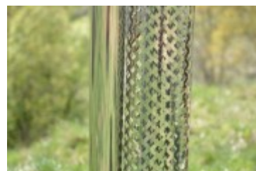
Metal safety fence for heater chimney
