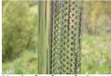
Metal safety fence for heater chimney
