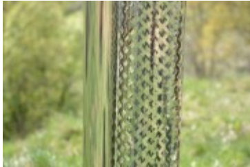
Metal safety fence for heater chimney
