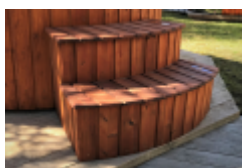
Stairs with niche for sand filter
