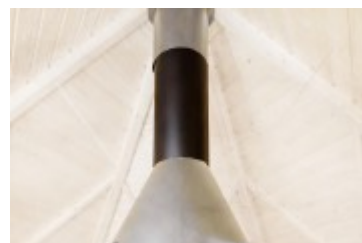
Grill Chimney Extension
