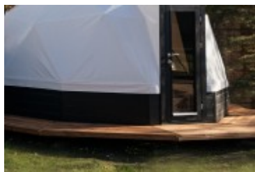
Terrace floor segments
